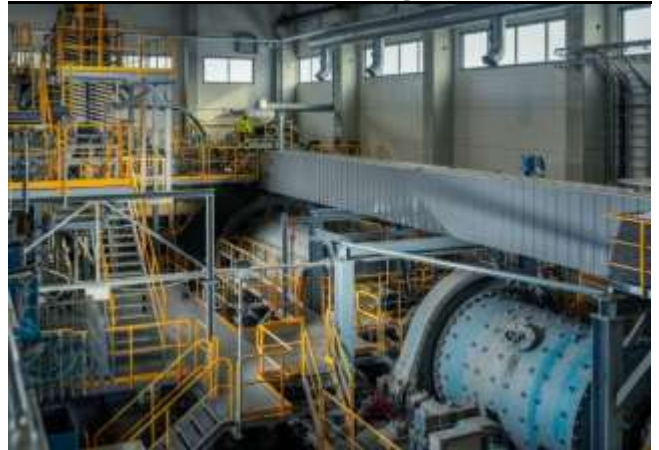
Inside view of the Pampalo processing plant
